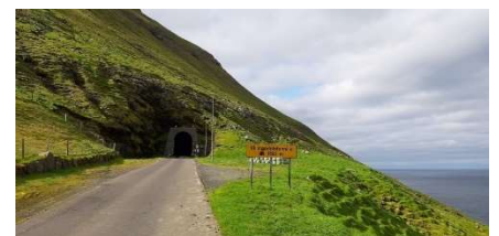
Tunnel op Kalsoy,
